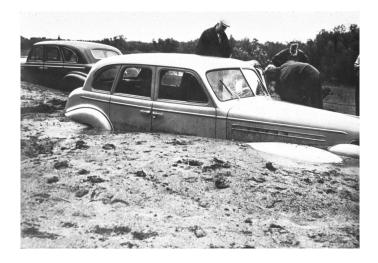
silt, and the once prosperous towns of Beaver and Whitewater Falls were eventually abandoned. Bridges were washed out and had to be repeatedly rebuilt, highway ditches and culverts became perpetually clogged with sediment and debris; repair and maintenance costs were out of control. Elba, which was once situated on high ground, survived only under the protection of dikes. Finally, in 1938 the Whitewater River flooded 28 times.
