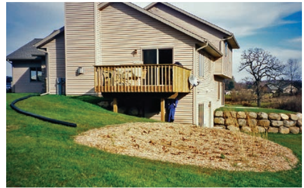
An extension of PVC pipe helps direct downspout water to this rain garden.
